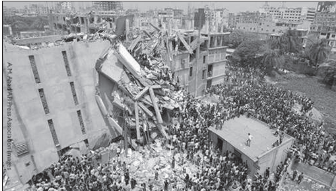
The collapsed Rana Plaza building in Dhaka. At PV press time, over 1200 bodies had been recovered from the rubble.
