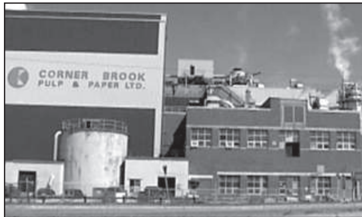
Kruger-owned pulp and paper mill in Corner Brook
