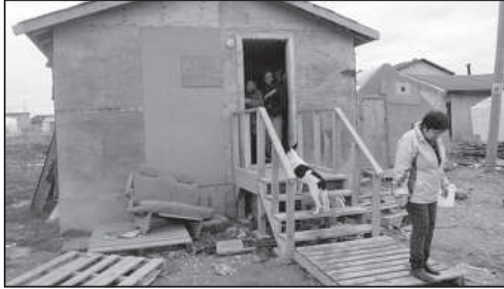
Deplorable housing on Attawapiskat First Nation
