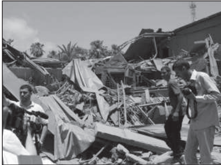
Damage caused by NATO bombing of Tripoli, June 2011
